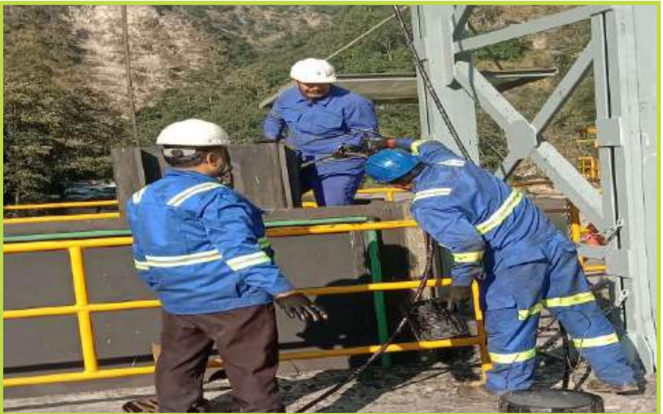
Under Sluice Bulk Head Gate Maintenance
