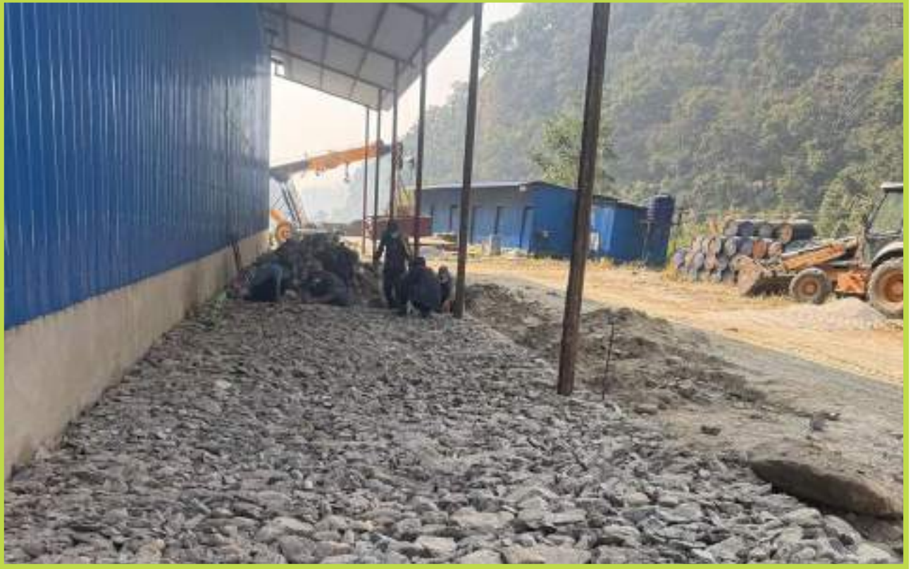
Main Store Extension
