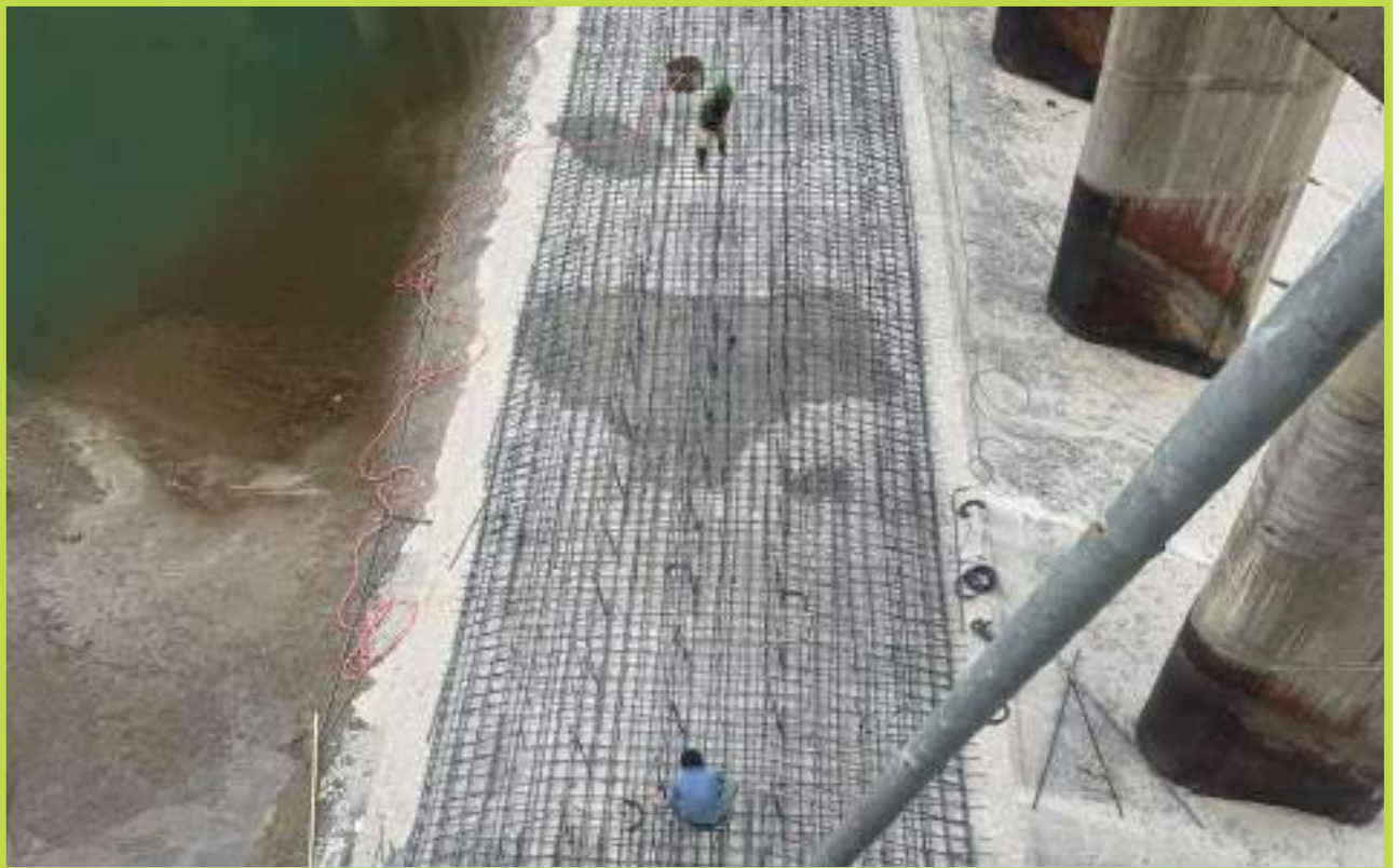
Reinforcement Work for Weir Crest Height Increase
