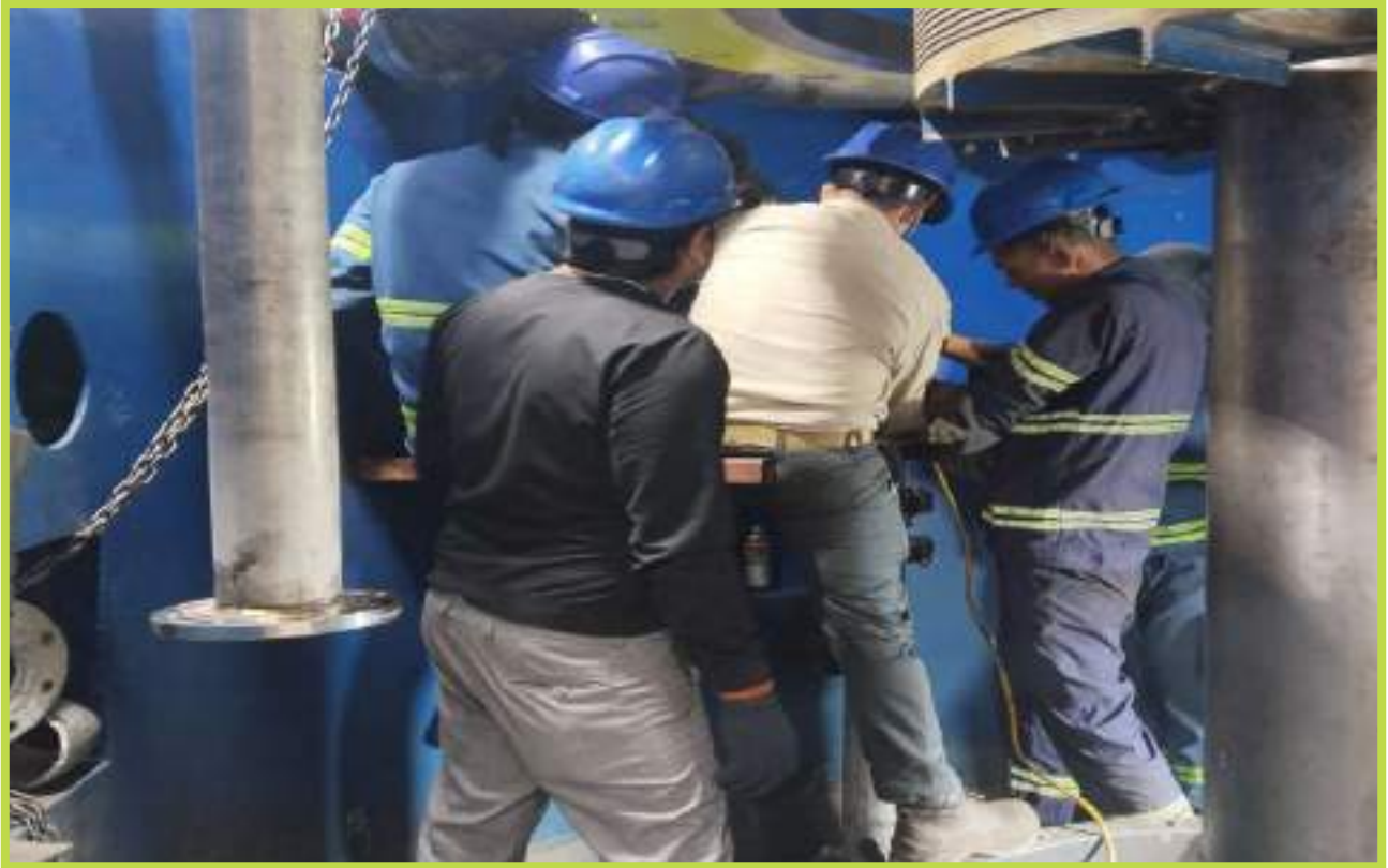
Balancing Pipe Installation
