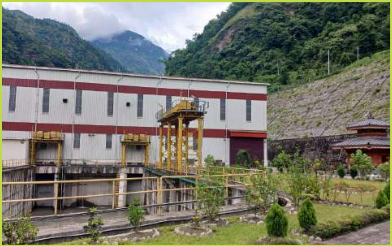
Power House With Tailrace
